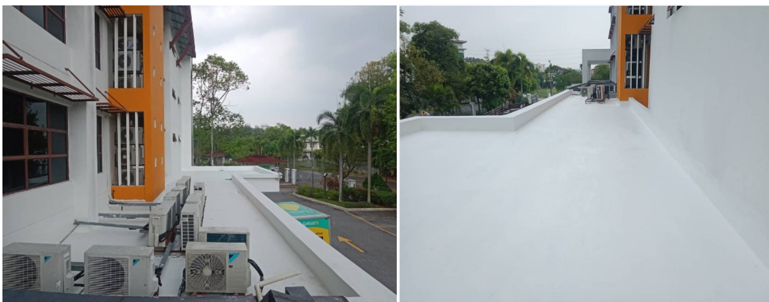
Concrte slabs Waterproofing in Australian international school
