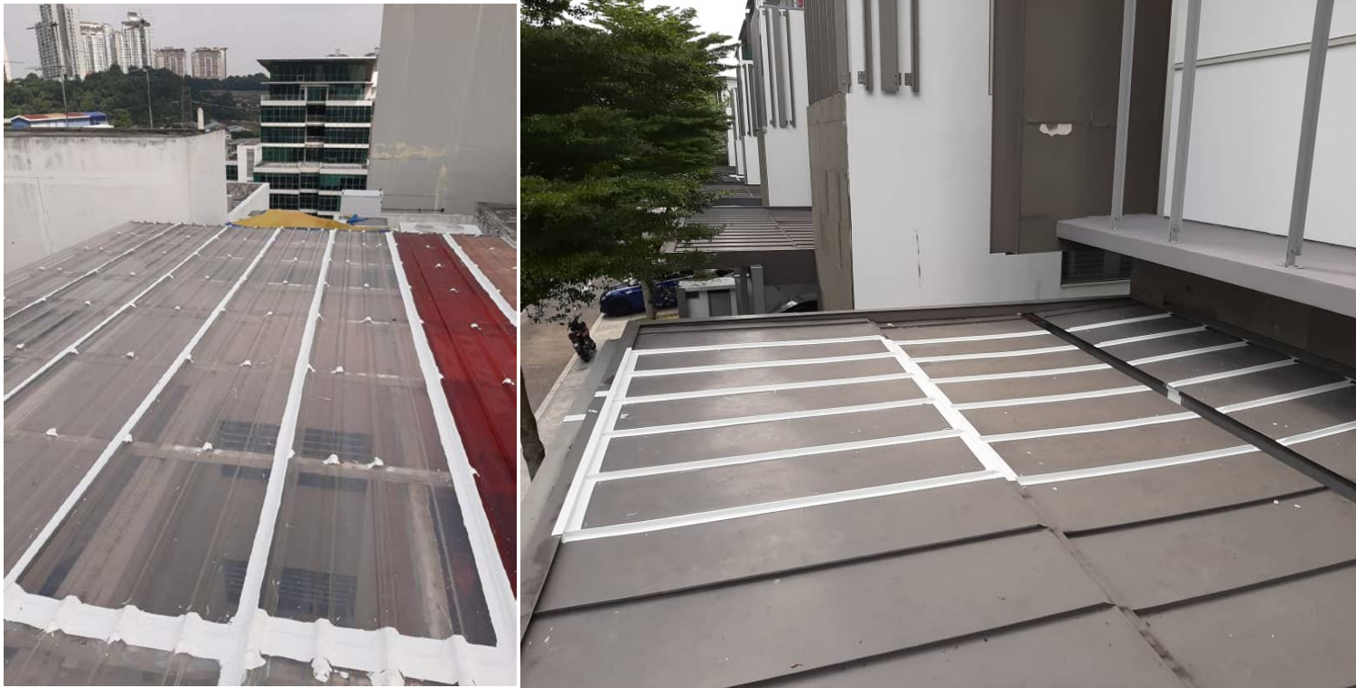
Metal and polycarbonate waterproofing in taylors university
